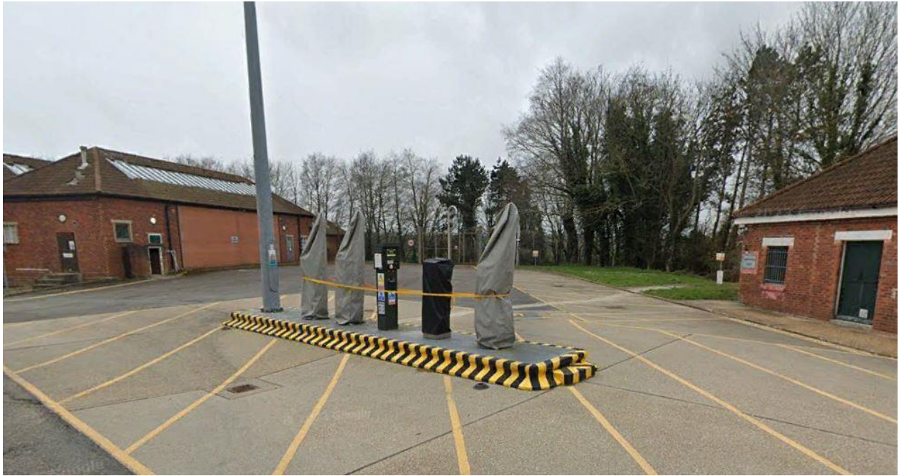
Plate 4. (Looking west over fuel pumps)
